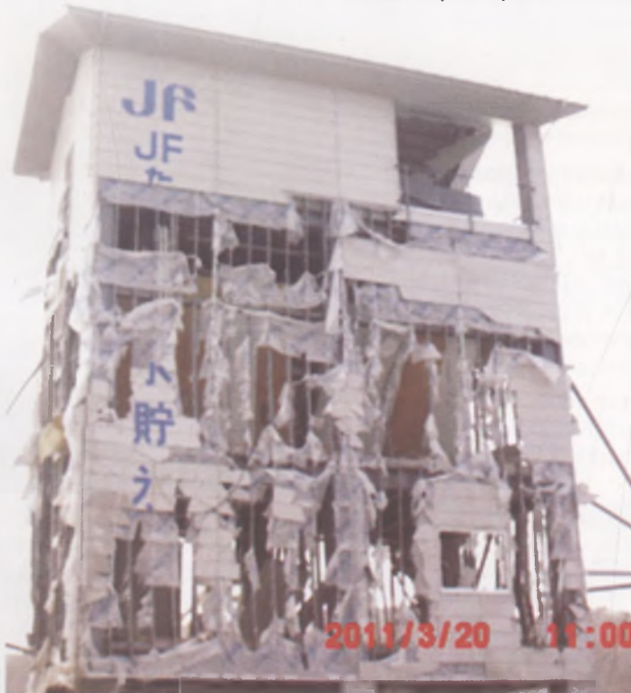
The ice-making facility of JF Taro FCA destroyed by the Tsunami
