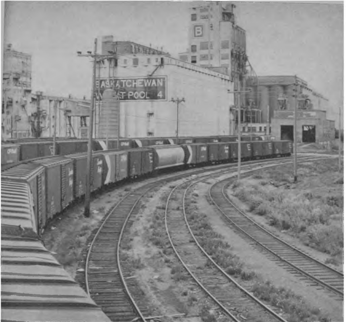
Saskatchewan Pool Terminal No. 4, Thunder Bay, Ontario.
