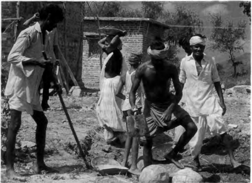
Self-help within the project Bonthapadu, India. Only local techniques are used
