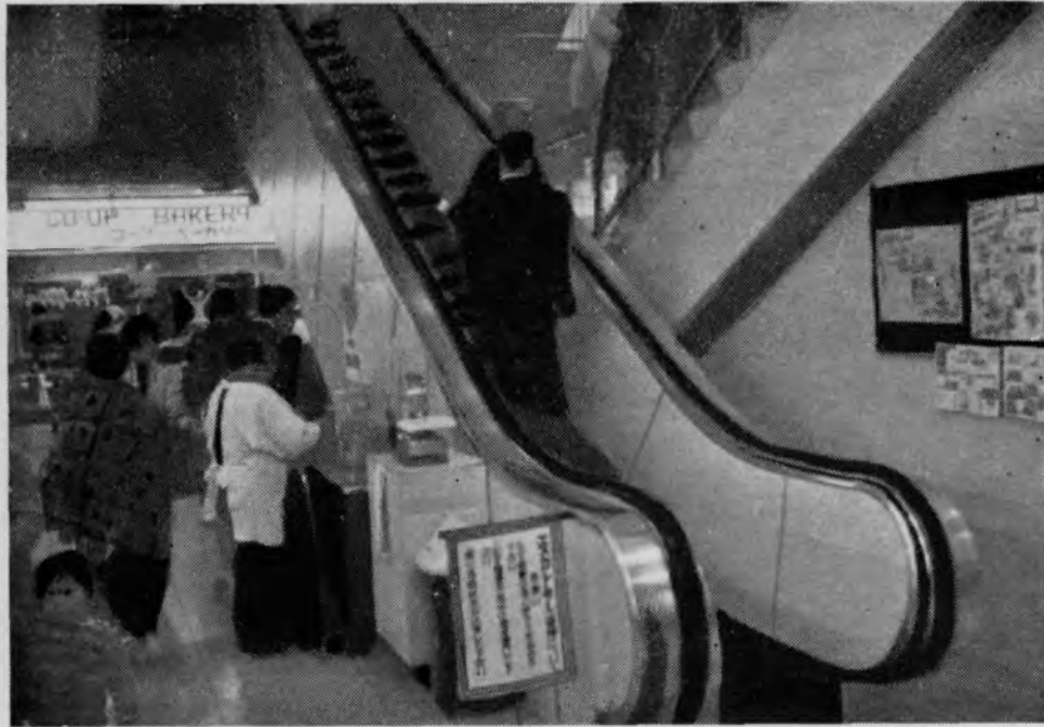
(xvii) Escalator helps flow of customers from one floor to another. This is commonly used in Supermarkets in Japan.
