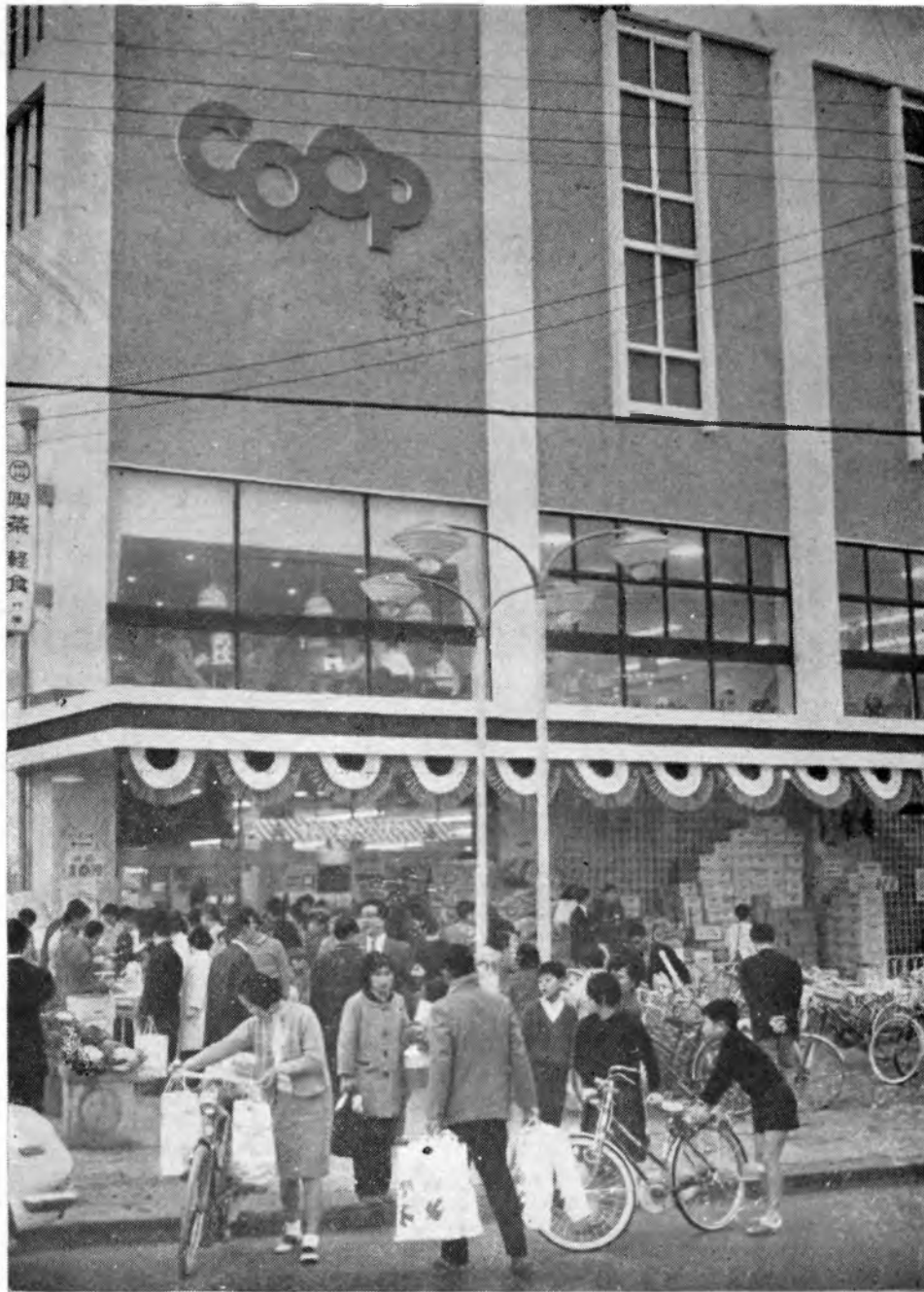
(xiv) A shop frontage in one of the cooperative stores in Japan. Note the symbol, spaciousness, cleanliness and smartness contributing to a proper image. The entire facade is designed to project the image of the store.
