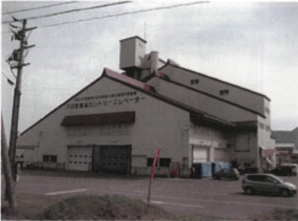
Country-Elevator, JA Uonuma-Minami
