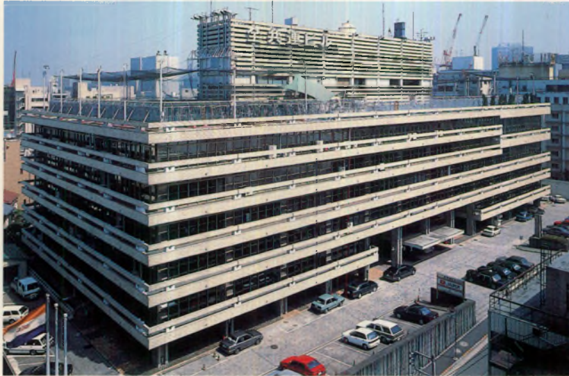
Zenkyoren Building, Tokyo
