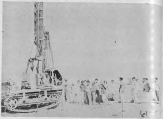
Members moving to action —tube-well drilling in progress in Barlai village.
