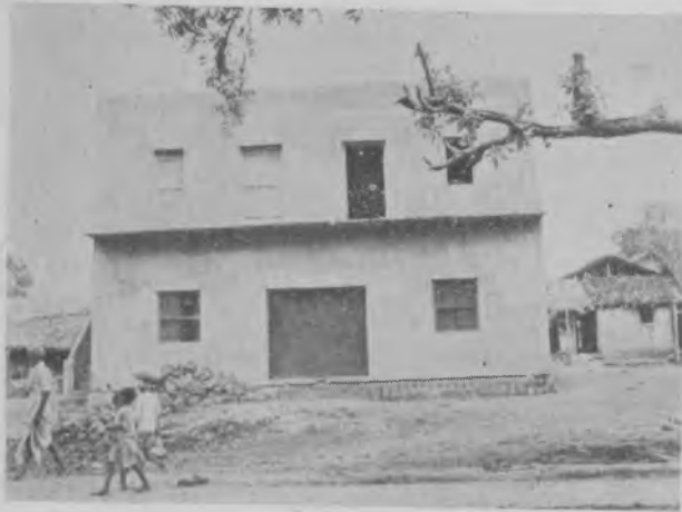
Newly constructed office-cum-warehouse of another society
