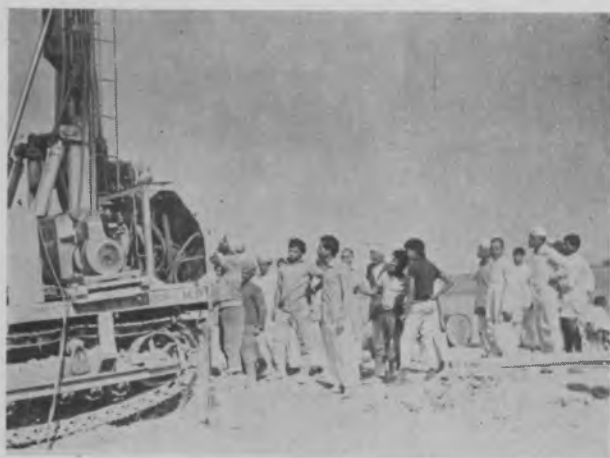
Tube-well drilling in progress in Barlai Village. Only 6.88% of farm land is under irrigation in the District
