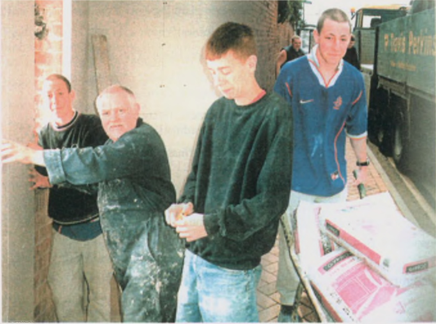
a. Skills training and Renovation Project in Wellingborough.
