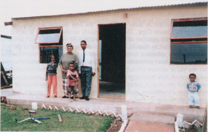
A family stands in front of their new, completed home, using the assisted self-help model. (photo: CHF)
