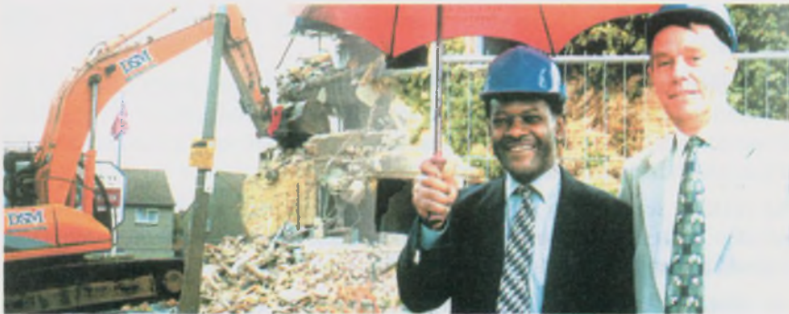
b. and c. Chairman of Foundation witnessing demolition of 'eyesore' flats.
