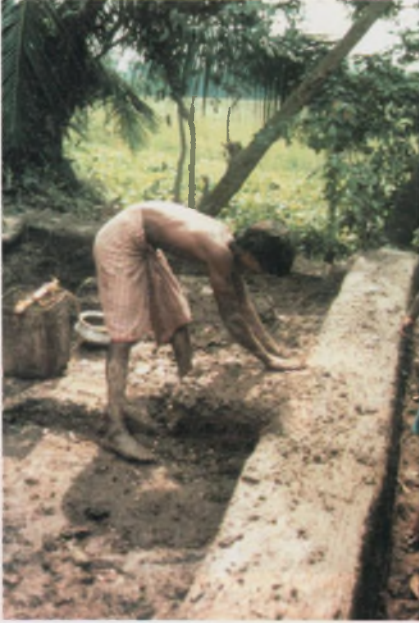
Avoiding waste of material: encircling it with blocks keeps the loose sand together. (photo: DESWOS)
