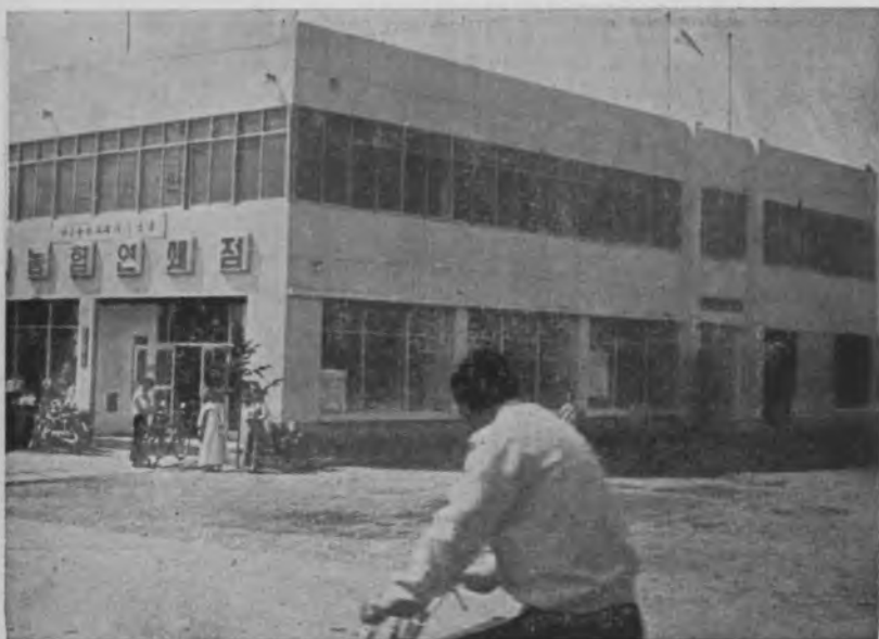
A newly constructed building of a primary agricultural cooperative society.
