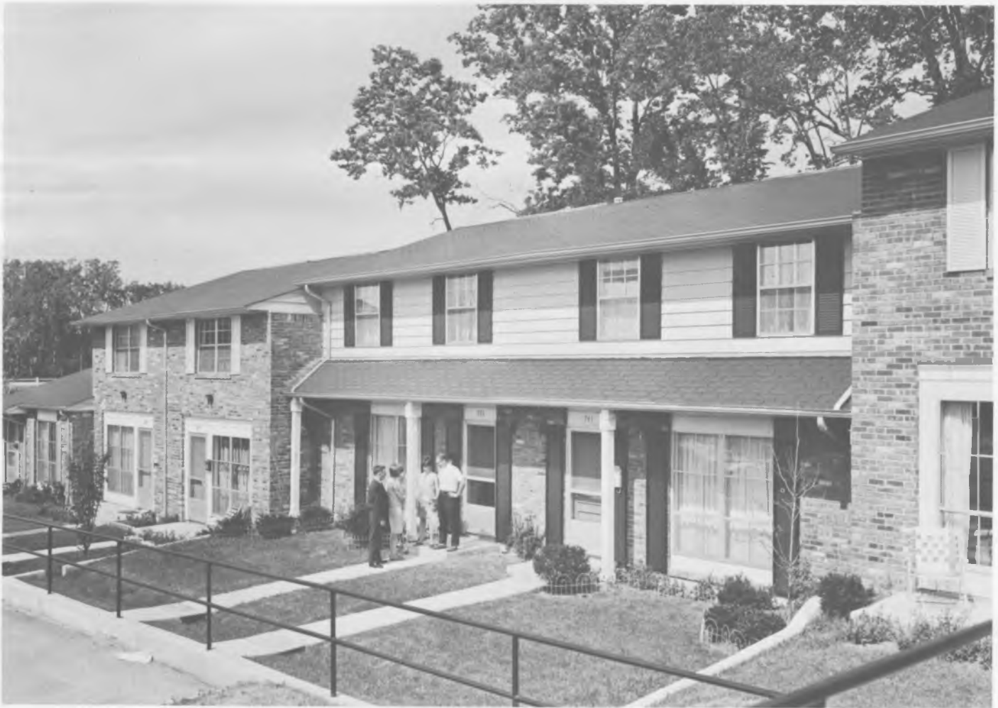
MODERATE-INCOME TOWNHOUSES built in Indianapolis for cooperative corporation using Federal programs convinced Gene B. Glick that because of economic necessity all housing for low and moderate-income families must be developed under subsidized programs in the future. Mr. Glick reports on how FHA Spec. 236 works in this accompanying article.
