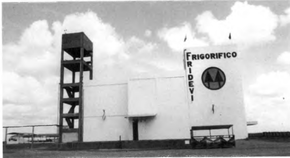
Fridevi - a cold storage plant for beef and lamb, located in Patagonia is another joint activity organized co-operatively between producers and consumers.
