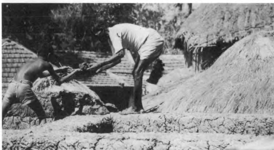
Mud construction in self-help housing.
