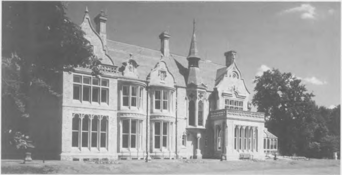
Denzell House, a period property of distinction in Altrincham, south of Manchester, houses the new ICMIF Secretariat.
