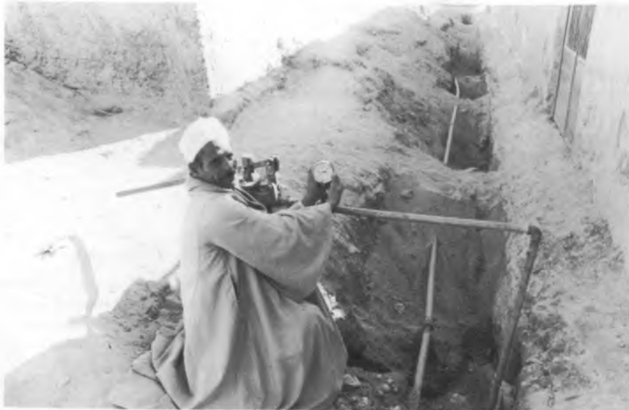
Below — AFTER: final solution — houses are individually connected to water supply
