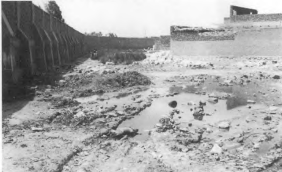
BEFORE: poor drainage, swampy conditions and cesspools (above)
