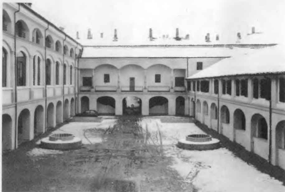
Co-op Casa di Cremona — An abandoned building is now residential apartments.
