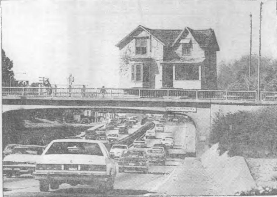
Why the House Crossed the Road ... Houses in the USA can be transported in one piece.
