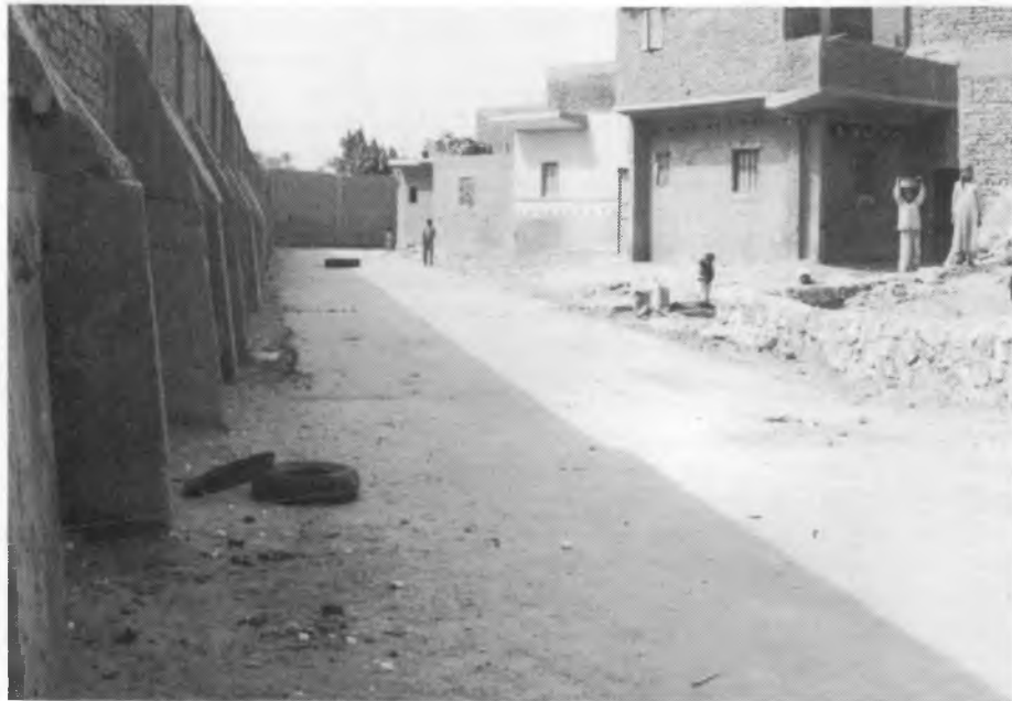
AFTER: construction of water and sewer network, road paving and solid waste collection programme, home improvements
