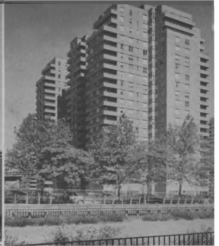
East River Housing Estate
