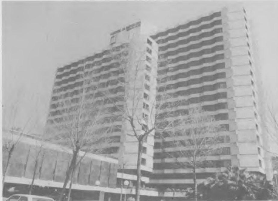
Solid efficient construction
