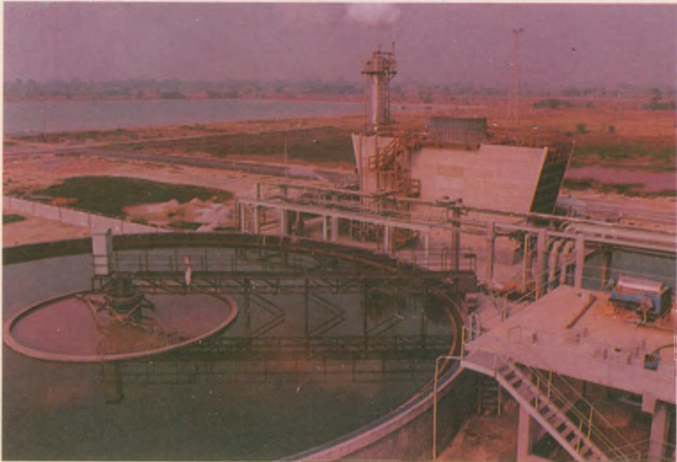
Centralised effluent treatment plant at one of the cooperative industrial units in India
