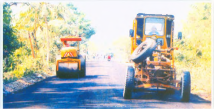
Road construction by Co-op
