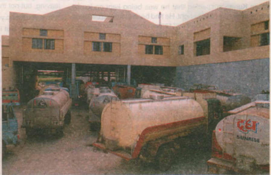
Milk being delivered to the plant in tankers - milk reception deck.
