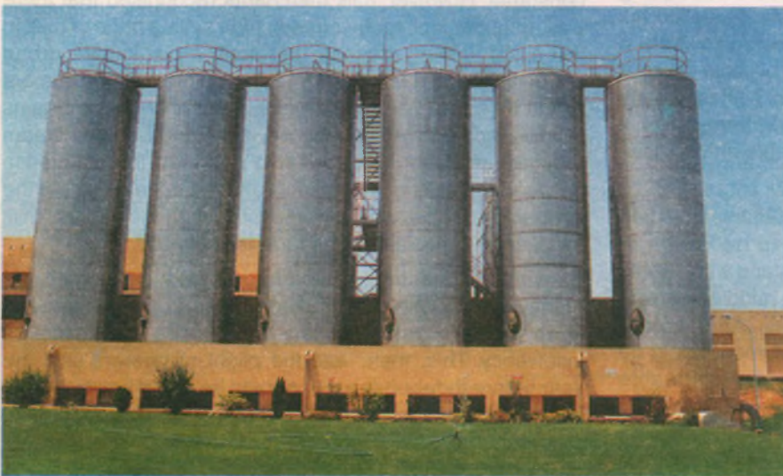
Mother Dairy storage tanks at Gandhi Nagar, Gujarat.
