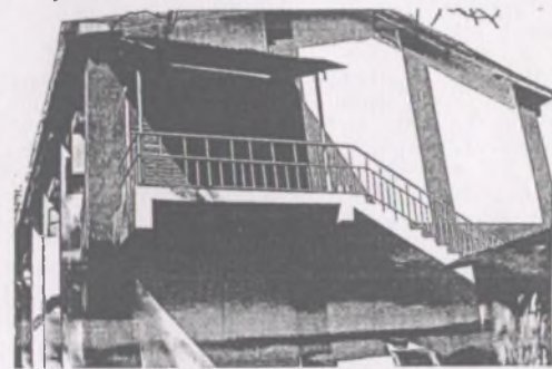
Post cyclone physical reconstruction of co-operative in Myanmar
