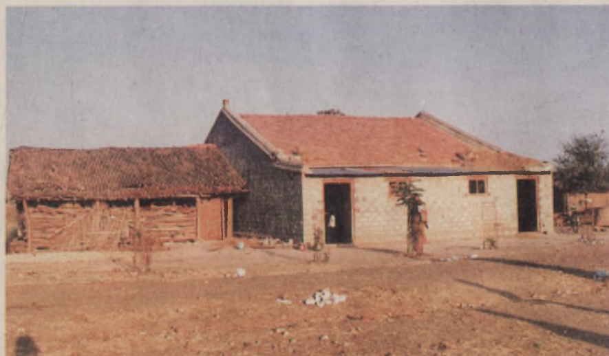
A house constructed under the Project
