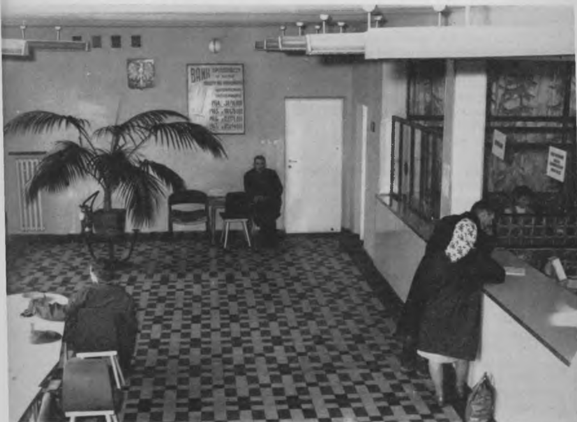
Interior of the office of the Co-operative Bank in Kutno
