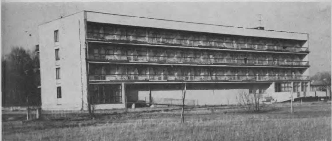
Sanatorium run by the Union of Co-operatives for the Disabled at the well-known watering-place of Busko-Zdrój
