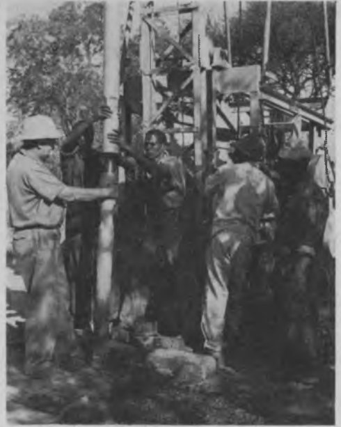
Boring for water
