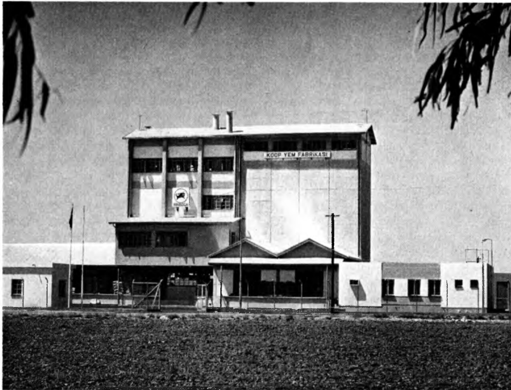
A compound fodder factory.
