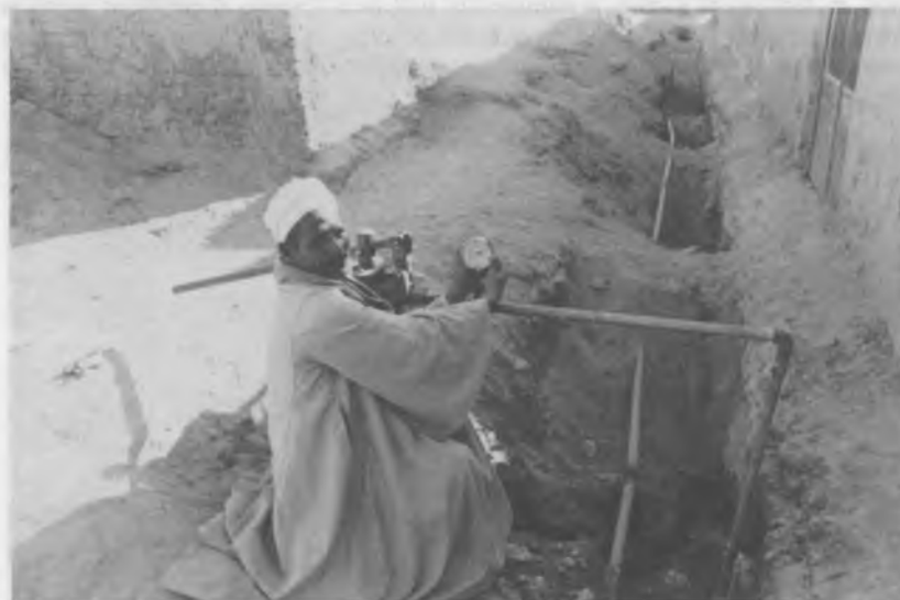
New water pipelines to the houses in Egypt
