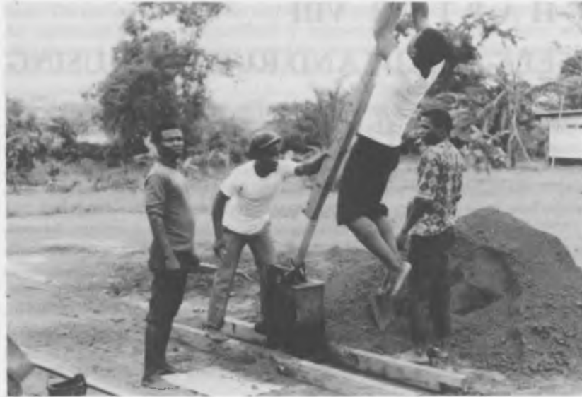
Project in Tema, Ghana: This Cinva Ram block-making machine can easily be used in self-help schemes
