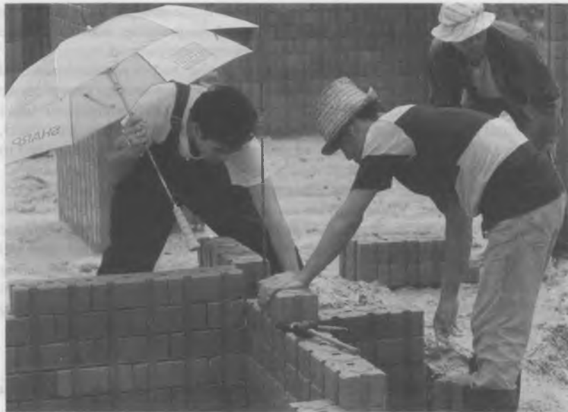
Self help in construction: The project of Ubon Ratchathani, Thailand A new laminated brick is being used
