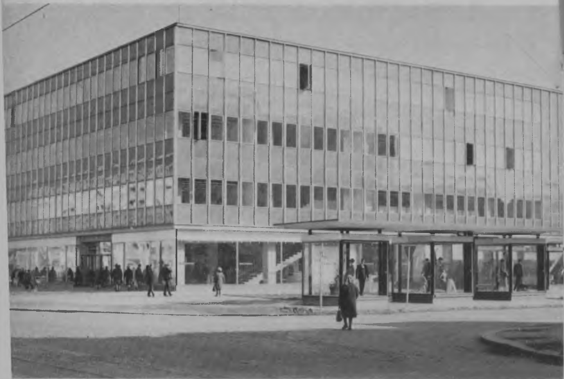
A new co-operative department store in Prague.
