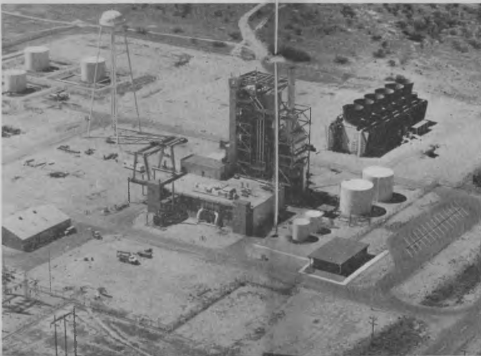
Arizona Electric Power Cooperative, which serves 50,000 members, recently opened this new power station at Benson.
