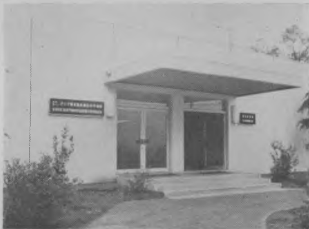
IDACA Building, Tokyo, Japan
