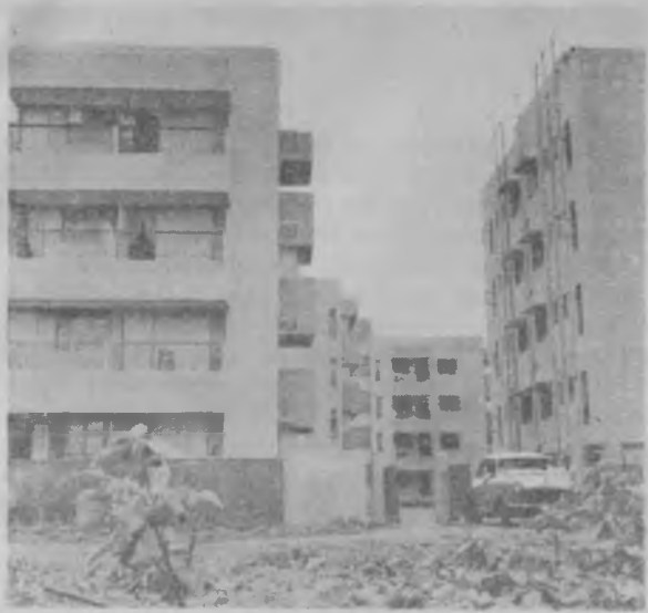
A housing project of the Bombay Dock Workers Co-operative in Bombay.
