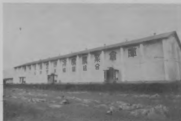
The society has several modern warehouses. This is one of them.
