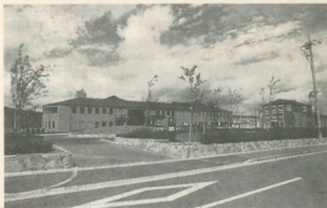
View of Seminar Building & Archive Building (right). Design of the Archive Building is modeled after the Rochdale Pioneers Museum in England
