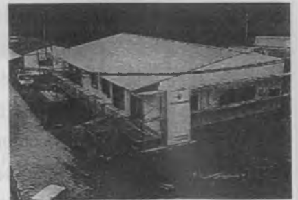
▲ Higashitsuru Plant Packaging Center
