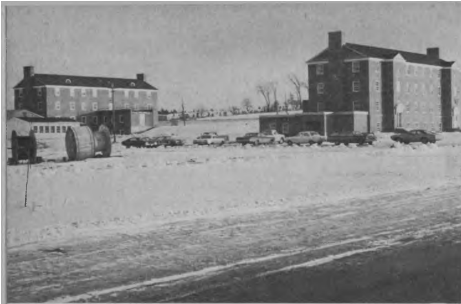
First Coady International Institute Residence and temporary classroom — auditorium and audio-visual training room (left), and second Residence Building
