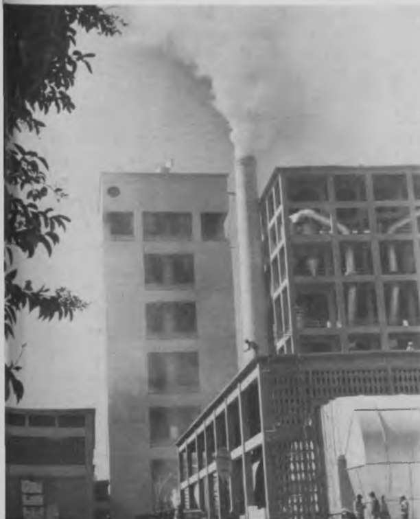
Electronically controlled Kilns of Cruz Azul Cooperative Cement Factory
