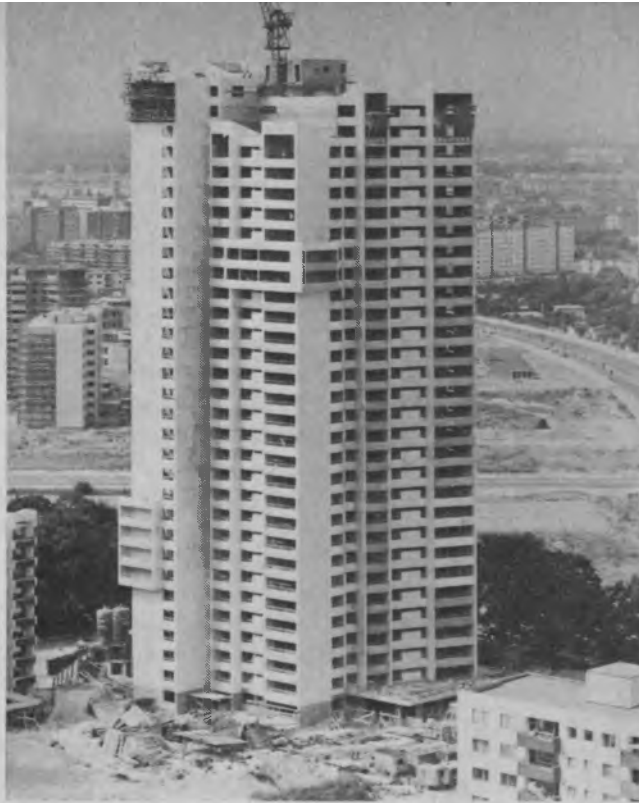
One of 30-storey sky-scraper blocks of Baugenossenschaft Ideal in Berlin, designed by Walter Gropius, as part of a housing project comprising 17,000 flats for about 60,000 people to be erected and completed in 1971 by 10 non-profit housing enterprises
