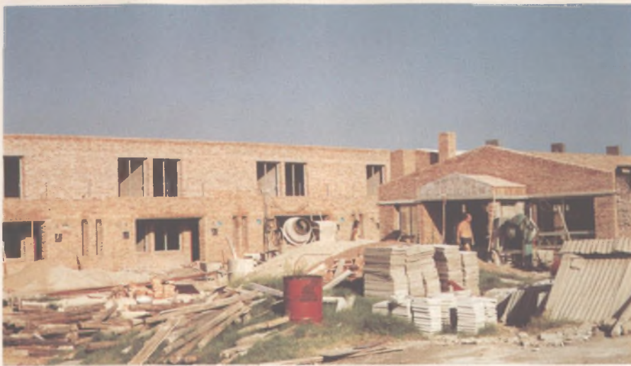
Co-operative/Municipality partnership leads to the re-housing of shanty town dwellers.
