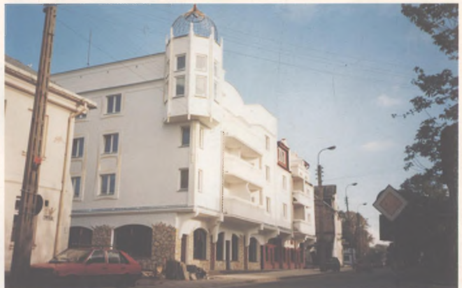
The Ulica Warszawska Co-operative Alternatywa of Bialystok, Poland, is a residential and commercial complex which symbolizes a dream come true for many residents and small business owners.
