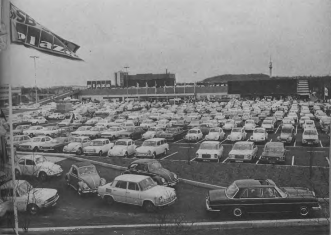
SB Plaza Department Store, Kiel
