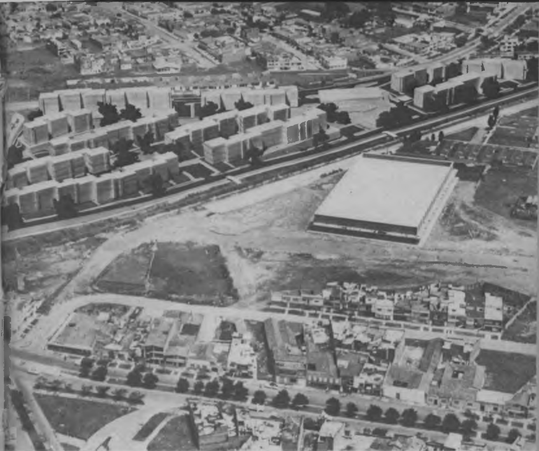
Co-operative housing project in Medellín, of 288 units
