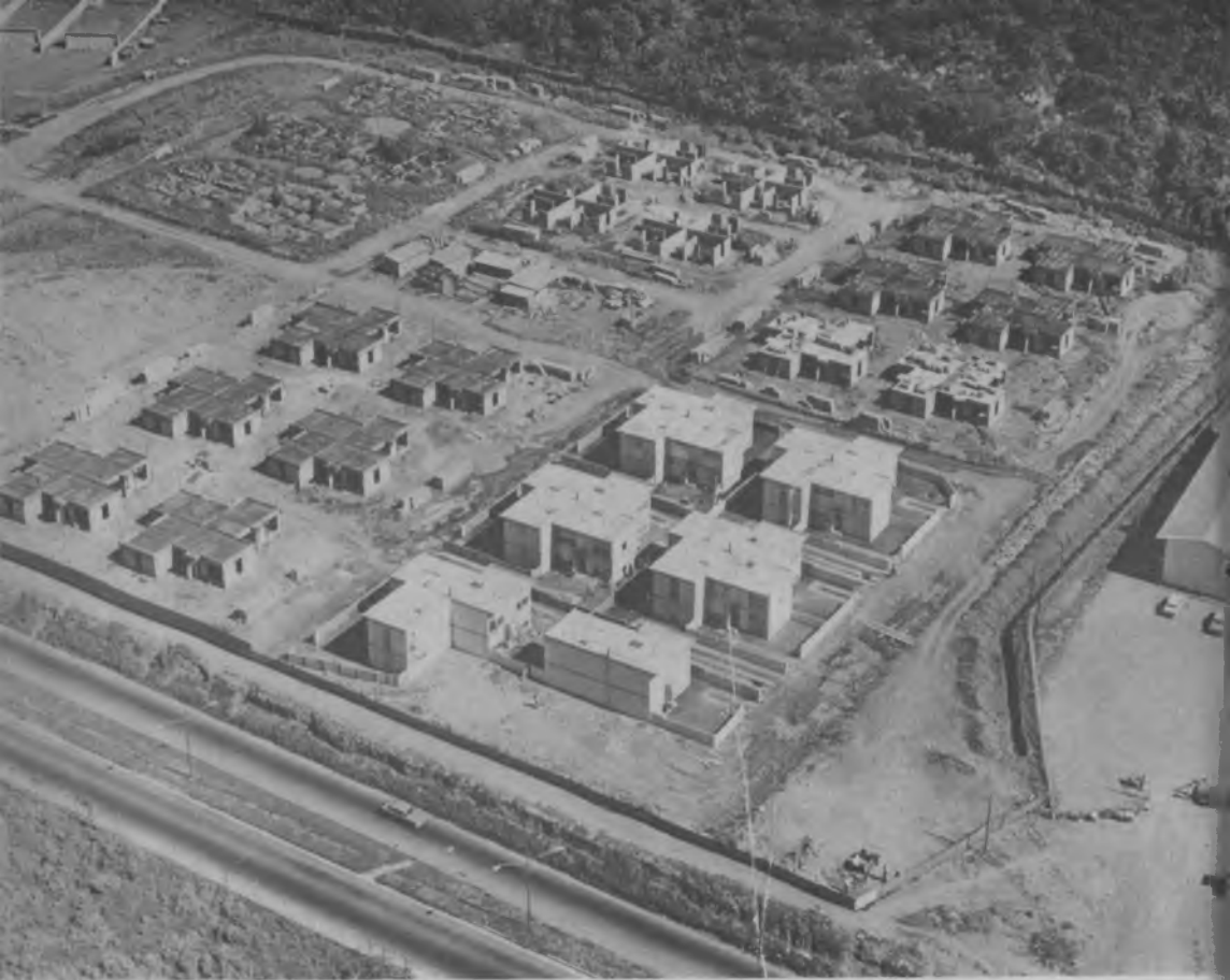
A Co-operative Housing Development which will include a primary school and community club (Jamaica).
