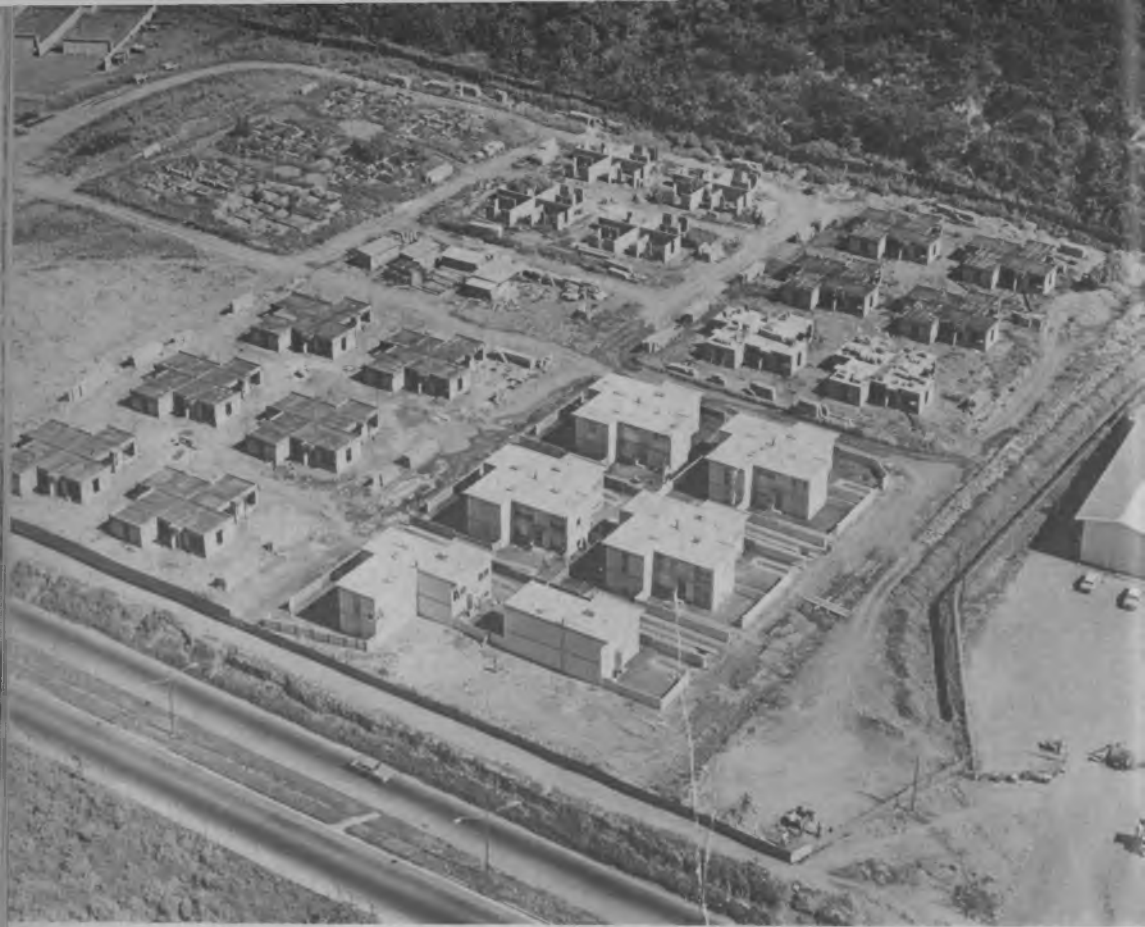
A Co-operative Housing Development which will include a primary school and community club (Jamaica).
