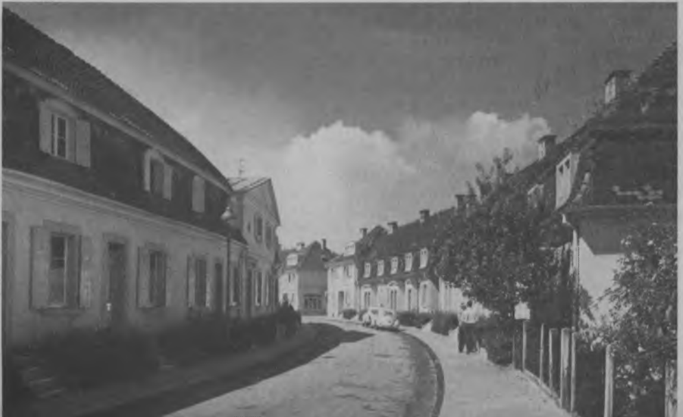
View of a terrace in the Garden City Estate, Mannheim, a cooperative project built in 1912
