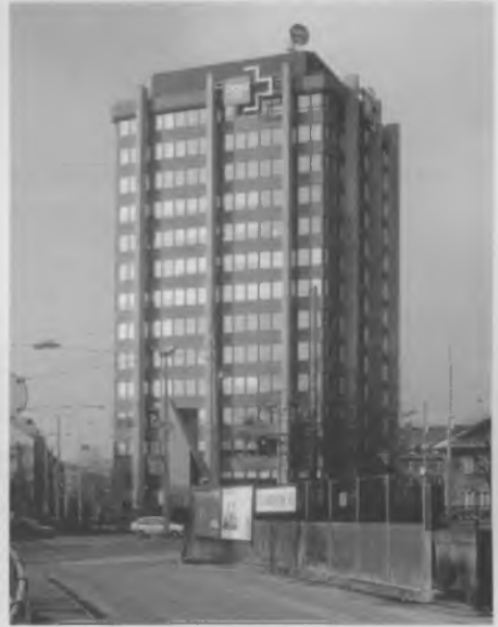
Co-op Switzerland's headquarters in Basle.
