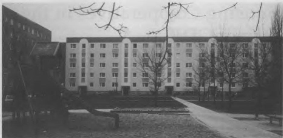
Rehabilitated inner court in a housing co-op in Eisenhüttenstadt.
