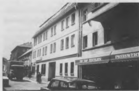
Two examples of projects from housing co-ops in the former GDR show high blocks with prefabricated elements in Magdeburg (above) and modernised old housing stock in Weida (below).
