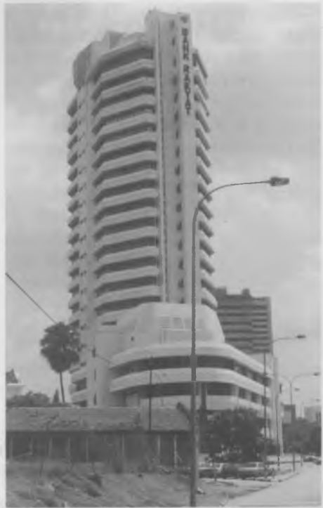
The People's Co-operative Bank stands in the centre of Kuala Lumpur, capital of Malaysia.
