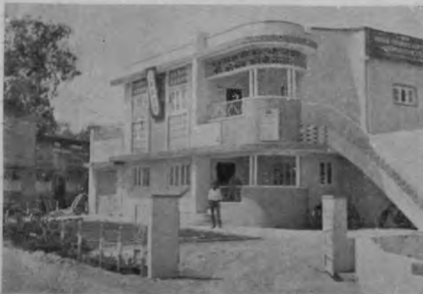
The Project Office
