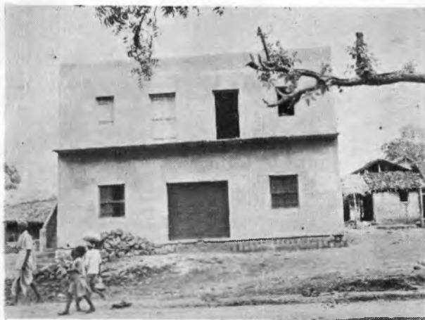
Newly constructed office-cum-warehouse of another society
